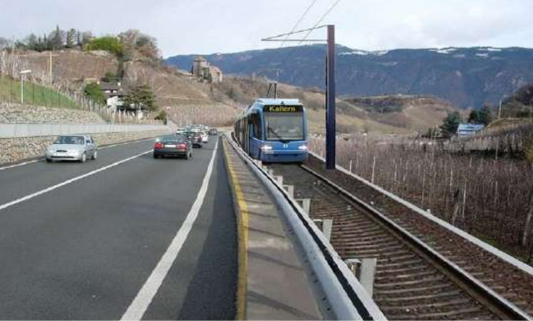
New tramway Bolzano – Caldaro
