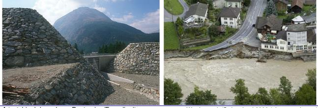
A 'catching' dam above Pontresina/Engadin; its construction became necessary when the permafrost area above the city began to melt. Cost: 5 million euros. (photo:GÖF)
