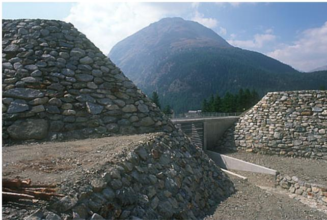
A 'catching' dam above Pontresina/Engadin; its construction became necessary when the permafrost area above the city began to melt. Cost: 5 million euros. (photo:GÖF)
