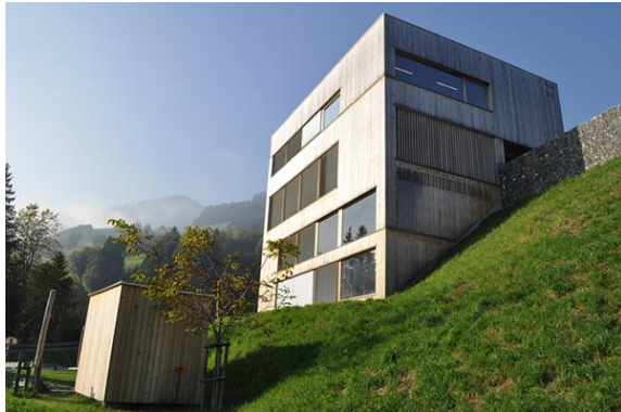
St. Gerold community centre – a modern, multifunctional building made of local wood. © Caroline Begle, CIPRA International
