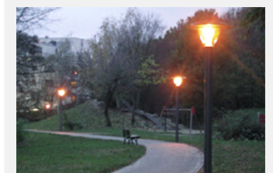
Solar lighting cuts down on costs and CO 2 .
